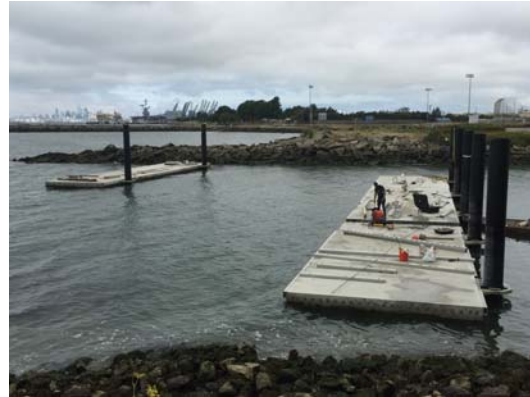
New wavemaze almost at completion
