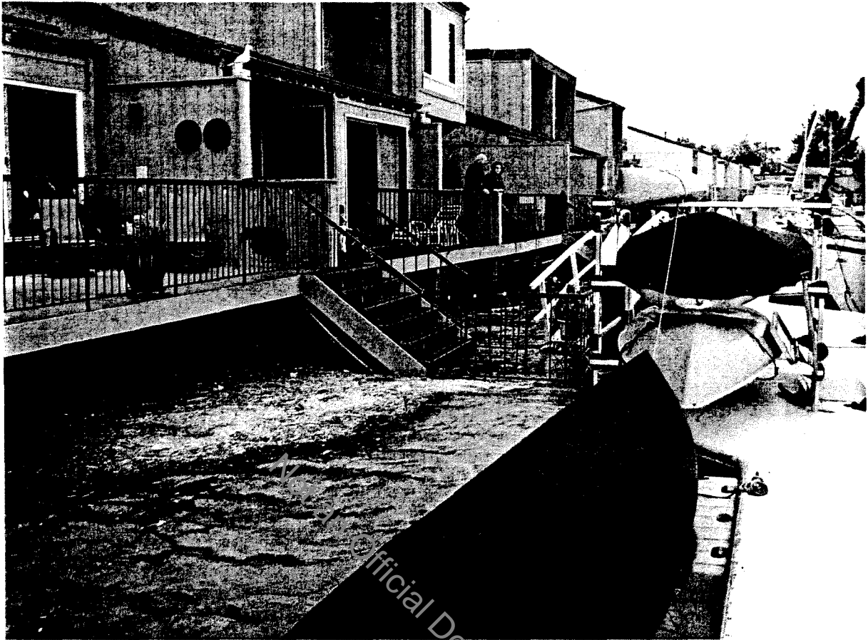
Storm waters flow over BBTA landings - December 31
